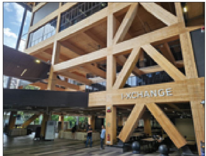
Mass timber was used to construct the ZEB and SLEB of BCA Academy Braddell campus.
